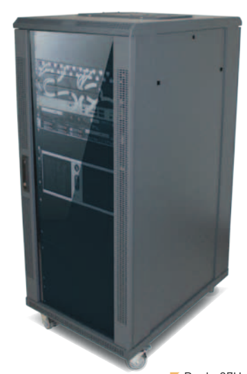
▶ Rack 27U (Mounted and adjusted)
